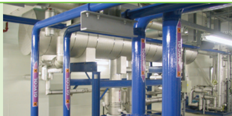
Plant room of a cold storage facility using carbon dioxide refrigerant (above and right)
