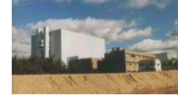
1993 Super GE (Super Conductive Electric Generator)
