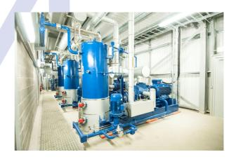
The bespoke refrigeration plant was designed to provide Yearsley Logistics with over 25 years of reliable service, with the lowest possible total lifecycle costs in terms of energy usage and maintenance. Star engineered and installed a single stage pump circulation plant, operating on natural ammonia refrigerant.
