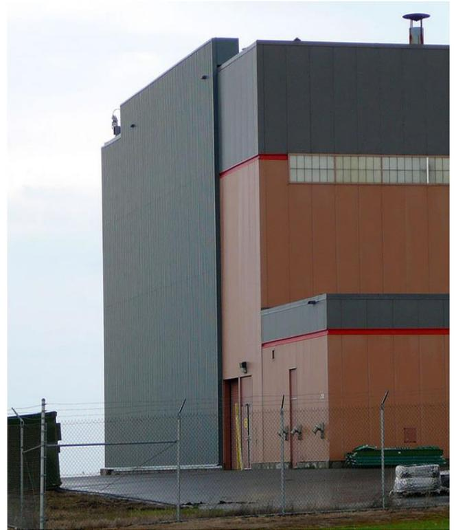
Solar air heating system vertically installed on exterior wall at Fort Drum, New York (Photo: Solar Wall).
