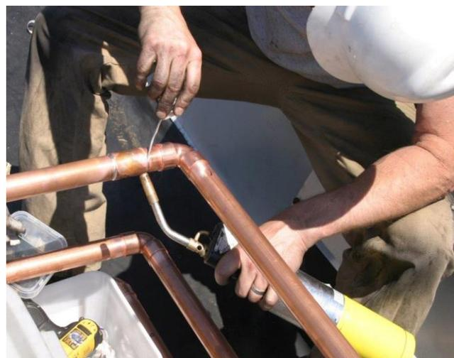
Copper pipes for circulating heating fluid through a collector are soldered together. (Photo: New England Solar Hot Water).
