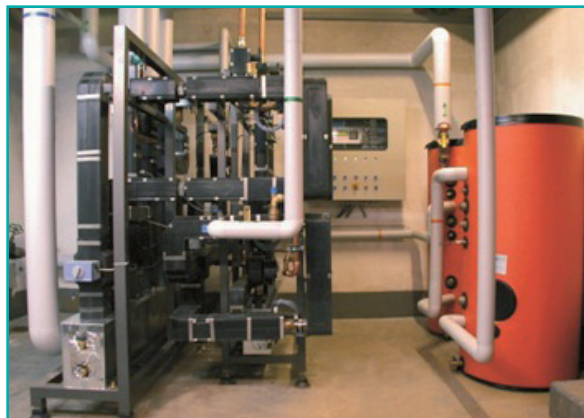
Figure 11 - Compact prefabricated hydraulic station for solar thermal systems in multi family homes. Source: Solvis.
